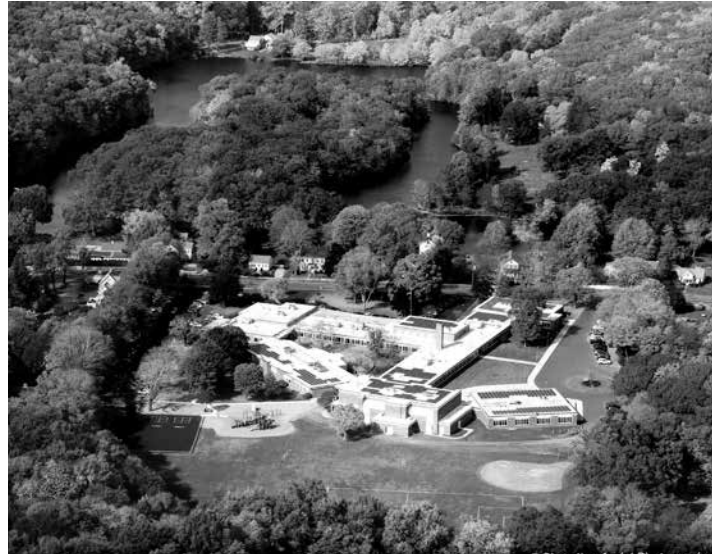
Aerial photo of the solar panel installation at Essex Elementary School. Photo by Shoreline Aerial Photography, LLC.
